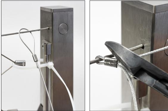
With installation rope 1,5mm (length at least 2 times post length) a very small loop is formed and pressed around the top tensioning rope.
