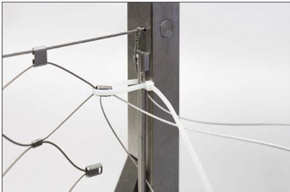
Make sure that a good tension is achieved at the end (correspondingly cable tie distance between clamps and round rod). Now you can cut off cable ties.
