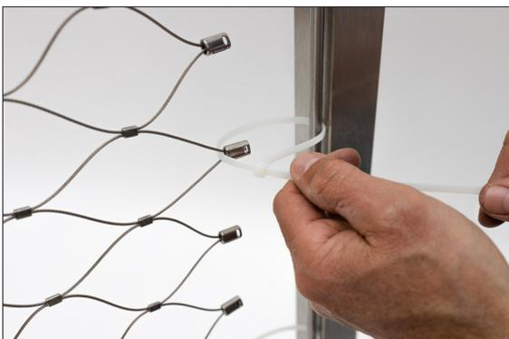
Cut the net direct at the net clamp. Install vertical rope clamps again and make the connection net with posts like the other side. Now you can adjust the desired und final tension with the cable ties.
